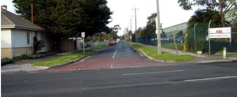
Coloured and raised pavement at Spotswood Primary
